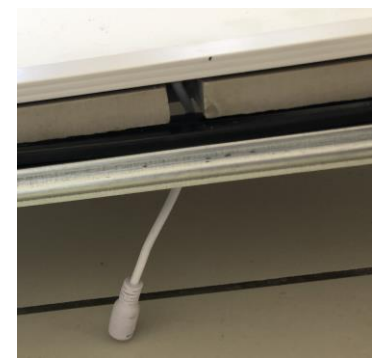
Fig 34 Example of slot for the electric wire
