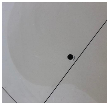
Fig 33 Example of hole for the electric wire
