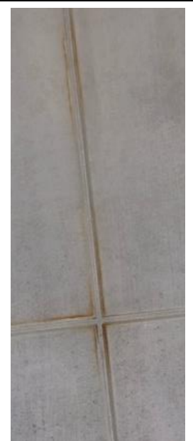
Fig 37 Example of contamination from tin
